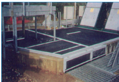
Covered (complex) Works Inlet
