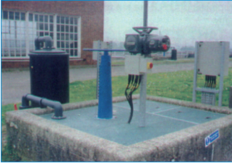
Typical Peackmaker 400 Module and Cover serving P.S.T. Well
