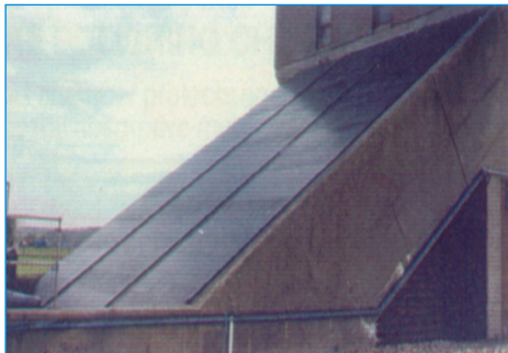
Covered Screw Pumps
