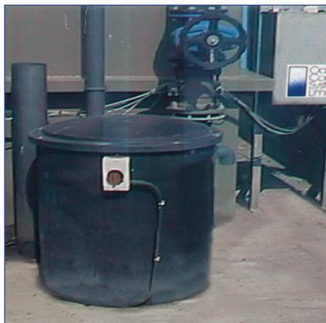
Foul air is drawn into the Peacemaker's inlet chamber and diffused via the lower diffuser which maximises its distribution across and through the dry impregnated media granules held in the odour oxidising chamber.
